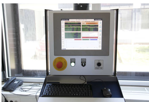
Figure 3.3: Control panel of the winding machine.
